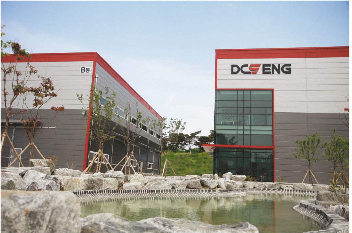
The picture of DCS ENG CO., LTD. main building
